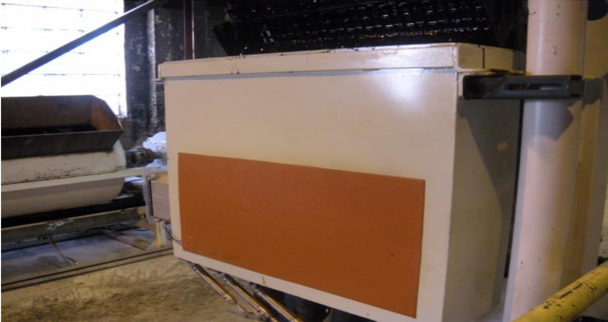
**(9) Clean Polished Bitumen Tank** – Bitumen from this tank is 99+% pure and ready for upgrading to produce Synthetic Crude Oil (SCO).
