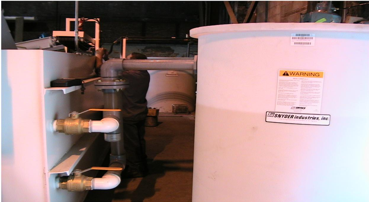
**(11) Surge Tank** – This tank holds the excess recyclable chemistry and acts as a buffer so as never to be short of process-ready chemistry.
